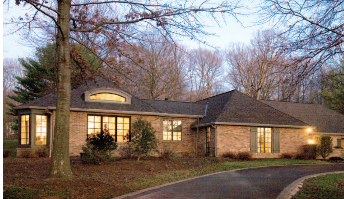
Matching the brick of the new addition to the existing house proved challenging, but worth the effort.
